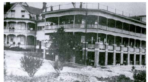
Figure 2.14 Shows the north and east facades of the 1920s Hospital addition which was named the Shannon Wing in the mid 1950s
