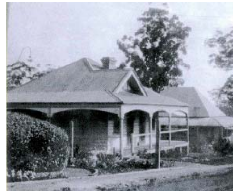
Figure 2.13 Undated photograph of "Bethel" House before the verandahs were enclosed
