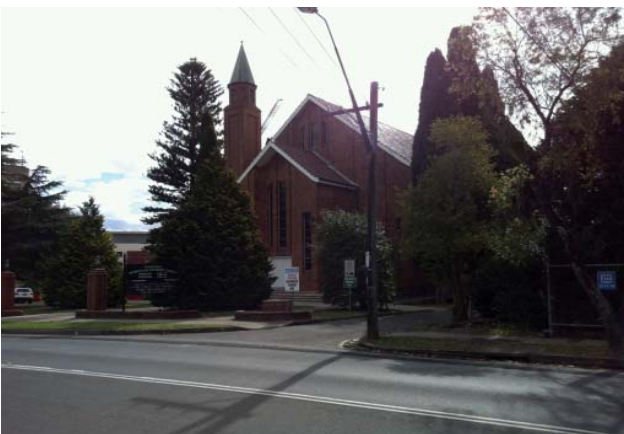
Figure 2.6 Seventh Day Adventist Church, immediately south of the subject site
