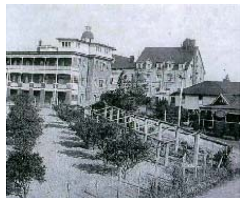
Figure 2.15 Shows the north and west facades of the 1920s Hospital addition. The roof level at the western end was removed at an unknown date
