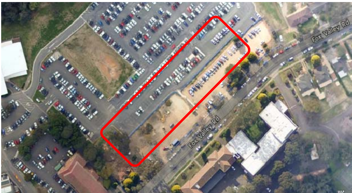
Figure 2: Area outlined in red shows post-demolition of former residential houses. The aerial image was taken in August 2012. (Aerial image source: Nearmap)
