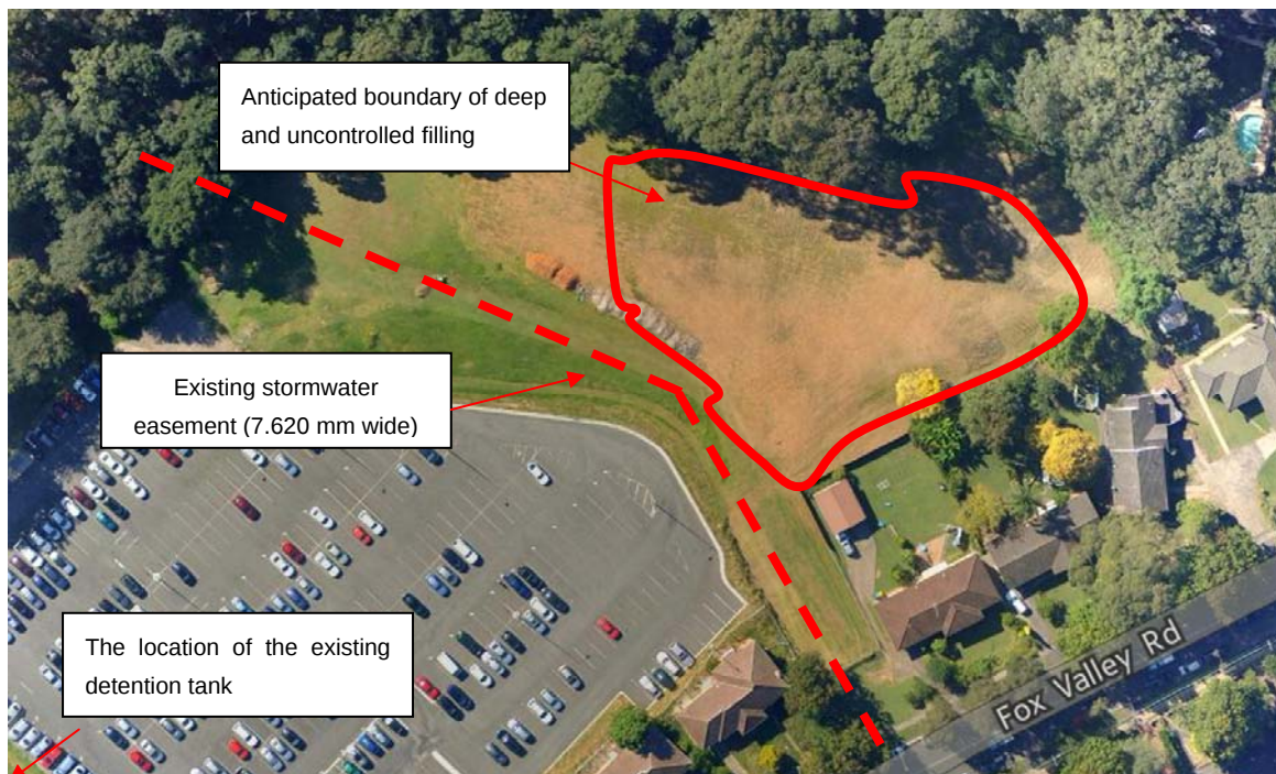
Figure 4: Area outlined in red marks the boundary of the anticipated boundary of deep and uncontrolled filling observed in the March 2012 aerial image. (Aerial image source: Nearmap)
