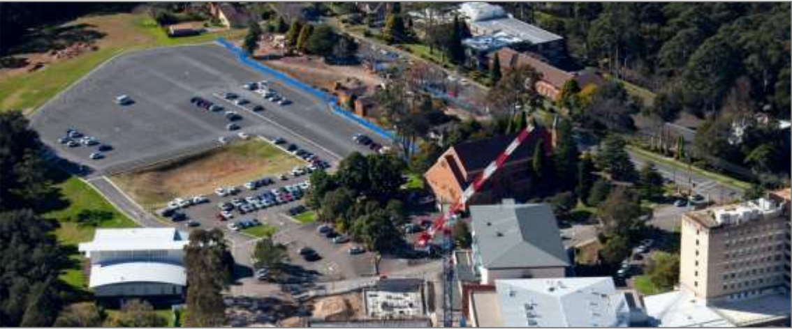
Site Image. Aerial looking north west
