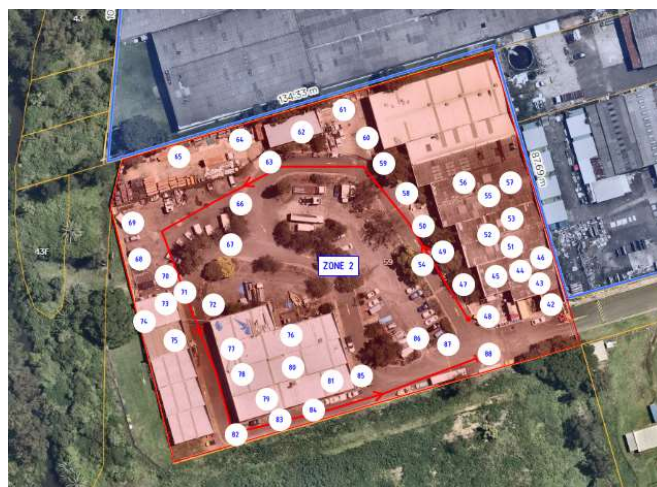
Image 5: Dilapidation survey for Zone 2
