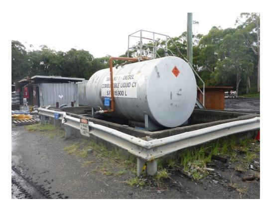
Photo 5 Diesel Tank stored within Bund
