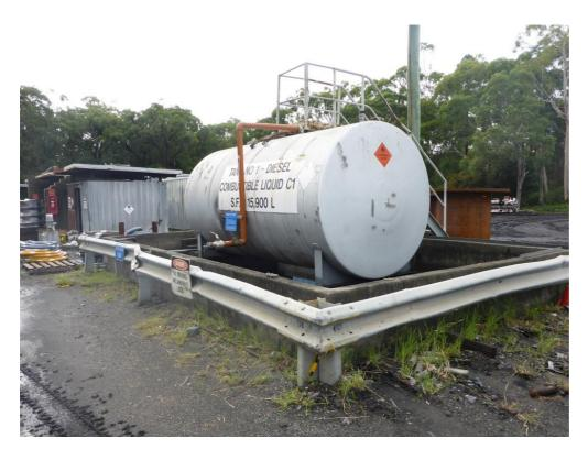
Photo 5 Diesel Tank stored within Bund
