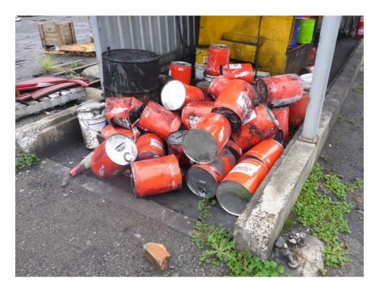
Photo 3 Hydraulic oil container stored on the side within bunded area. Improvement Required.
