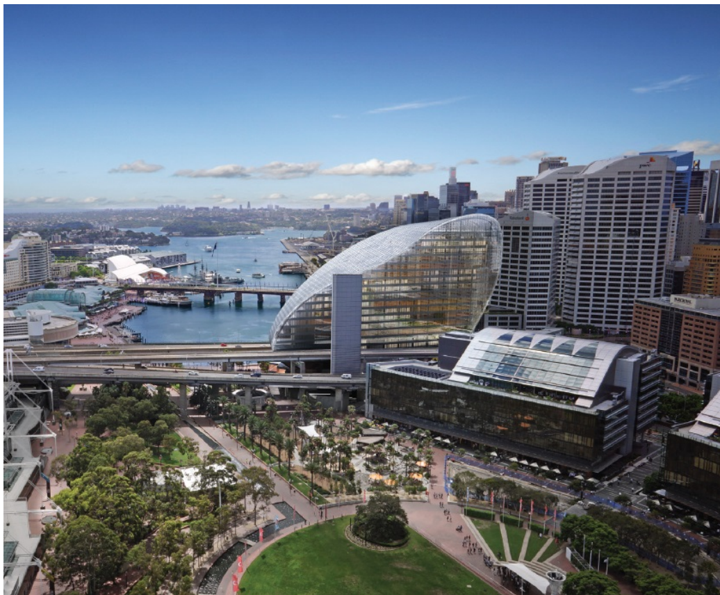
Figure 2. Proposed IMAX building with Tumbalong Park and Darling Quarter foreground Source: Proponent's SSD Application
