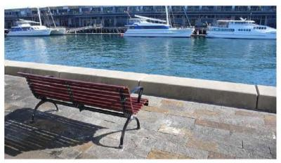
MATERIAL: AUSTRALIAN PORPHYRY PAVERS SIZE: 140MM SAW CUT WIDTH, 200MM/320MM RANDOM LENGTH SPUT ENDS FINISH: NATURAL CLEFT TOP SURFACE INSTALLATION: CEMENT STABILIZED SAND SETTING GED
