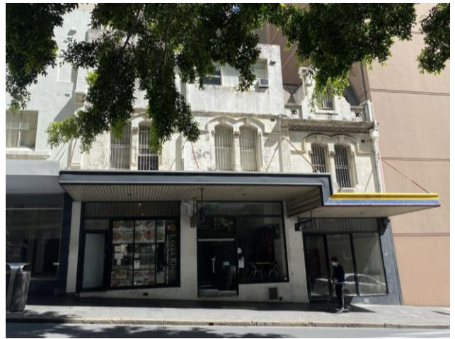
Picture 4 – Existing Commercial Terraces at 35-39 Erskine Street (Facing South Source: Urbis (2022))
