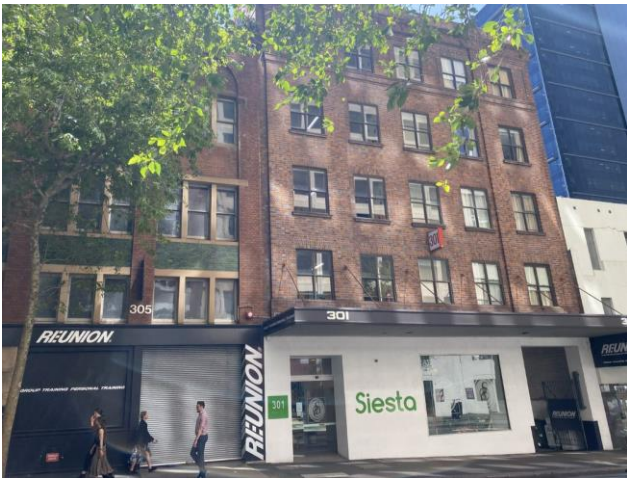
Picture 3 – Existing Buildings at 301 and 305 Kent Street (Facing West) Source: Urbis (2022)
