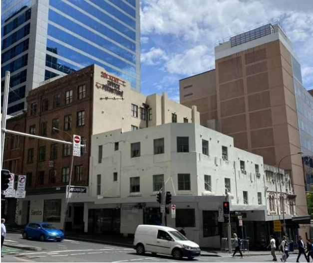
Picture 1 – Existing Development at 41-45 Erskine Street (Facing Southwest)
