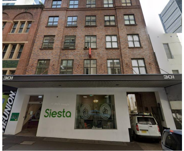
Picture 2 – Existing Building at 301 Kent Street (Facing West), including Right of Way
