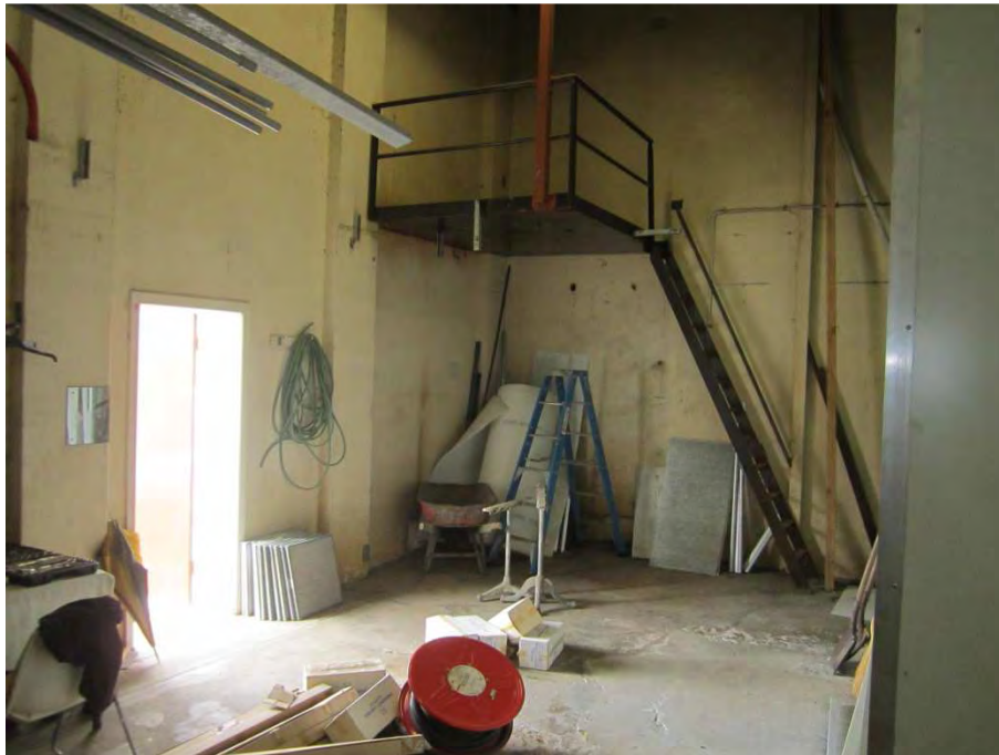
Photograph 1, Photograph shows the southeast corner of the former boiler building.
