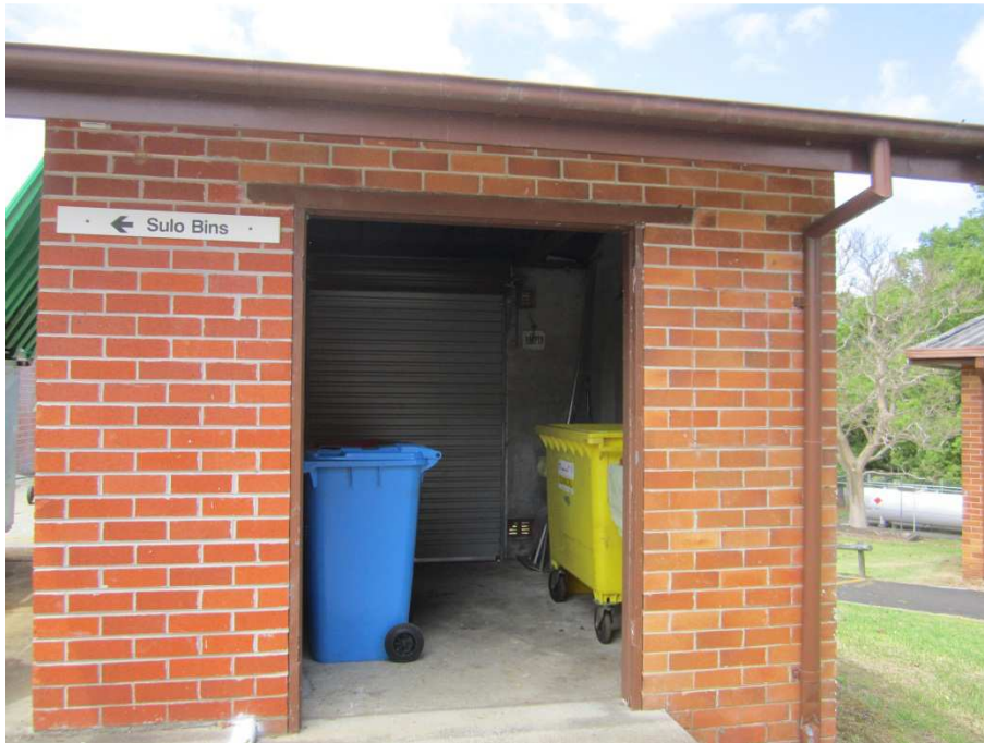
Photograph 5, Photograph shows the former coke storage building, now currently used for storing bins.
