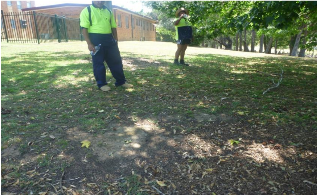
Plate 1: Kempsey District Hospital eastern portion, example of exposure, looking north.
