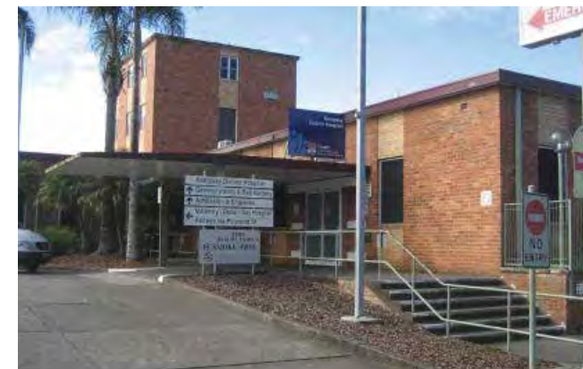
Emergency / Theatre Block
