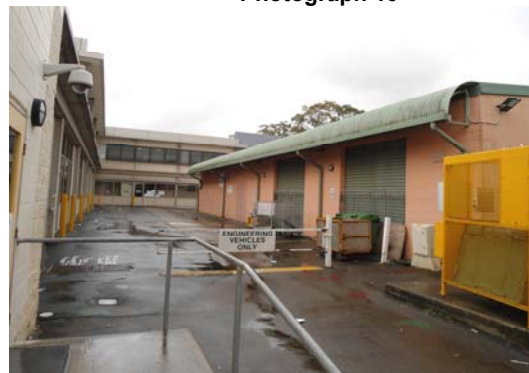
Maintenance Workshop Building
