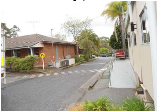
Driveway from Derby Road and Staff Cafeteria Building
