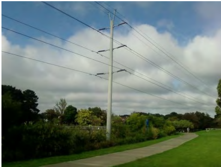
Figure 3.3 Example on left of spun concrete poles and wires (image provided by AGL)
