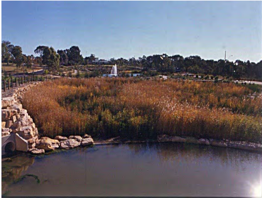
PLATE 6.4 CONSTRUCTED WETLAND (FOREBAY, MARSH AND OPEN POND)
