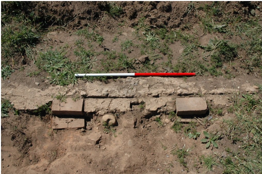
Figure 2.6: The mixed concrete footing with two stepped brick pads. Scale 1m. C&L2012.
