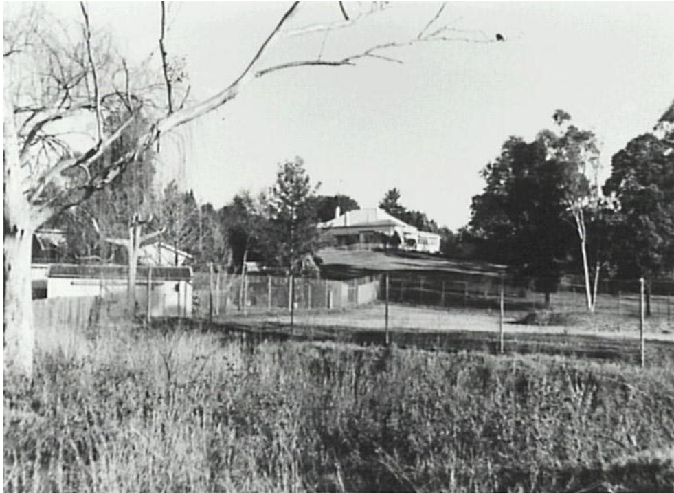
Plate 2. View of Thornton Hall in 1986 showing the localised high point (Penrith City Library)
