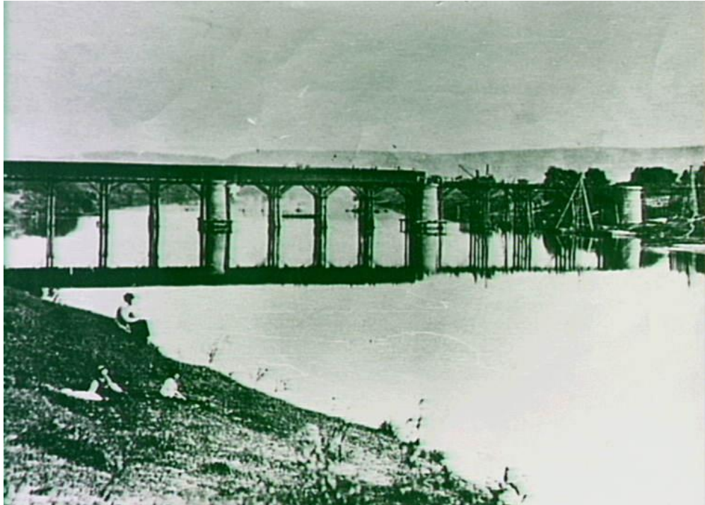
Plate 1. Photograph of the construction of Victoria Bridge c. 1865 (Penrith City Library)
