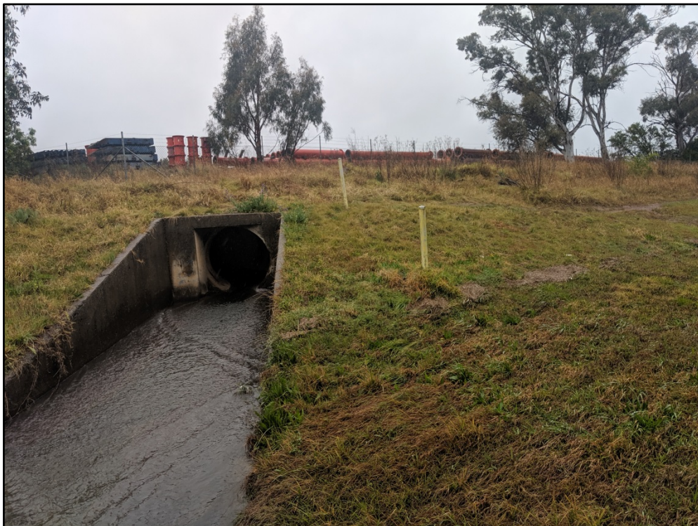
Photograph 20: Looking south-east at a stormwater pipe in the foreground, inferred to run between the exterior northern boundary of the site, through an alley. The north-western boundary of the site can be seen in the background (18 September, 2019).
