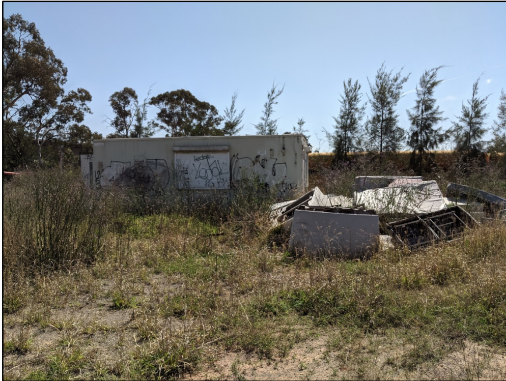
Photograph 11: A dilapidated site shed located in the southern half of the site. A small accumulation of mattresses, gas canisters and general rubbish can be seen in the foreground (4 October, 2019).
