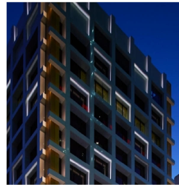
WINDOW FRAME LIGHTING, HIGHLIGHTING OPENINGS.
