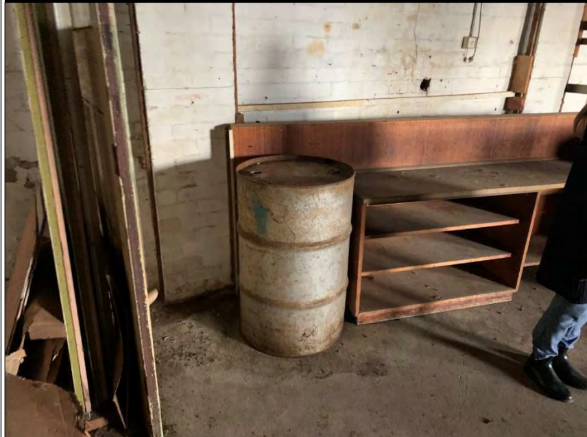
EMPTY DRUM IN BUILDING B
