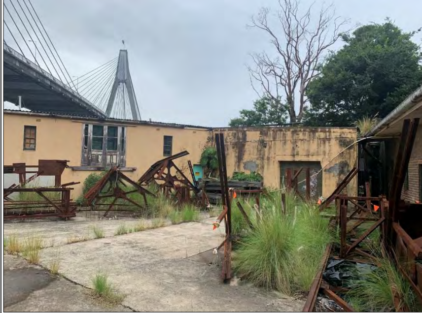
NORTHERN PORTION BUILDINGS AND REMNANTS OF COAL LOADERS
