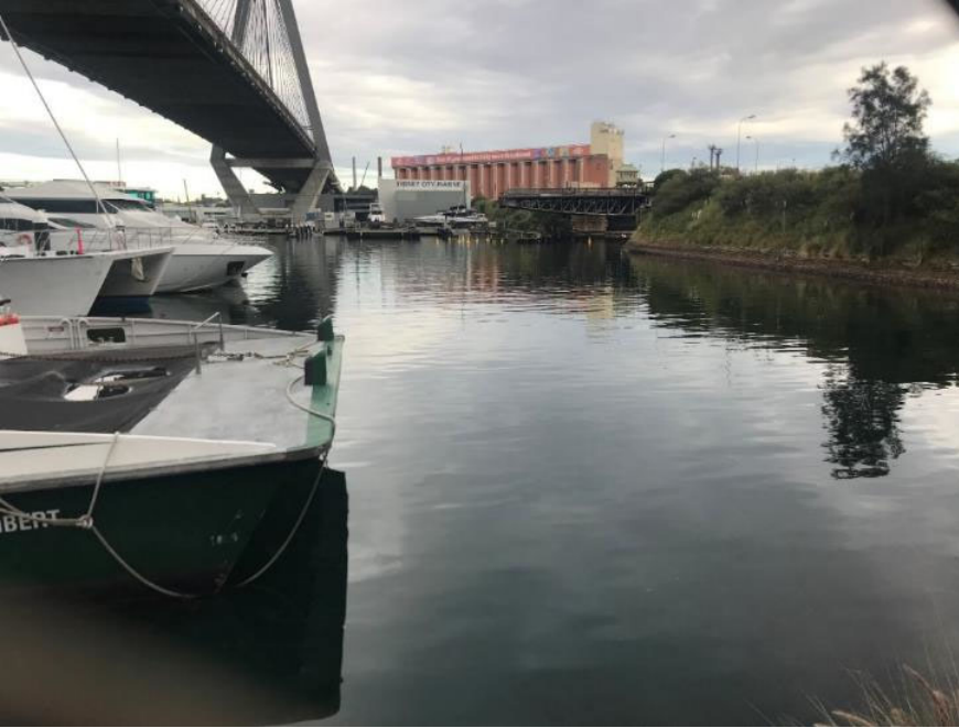
Figure 3.6 View of Glebe Island Bridge
