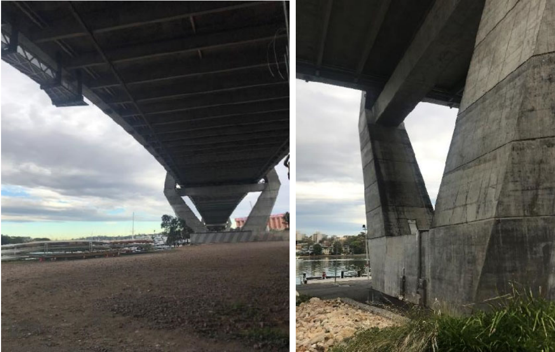
Figure 3.7 View underneath Anzac Bridge / Anzac Bridge Pylon
