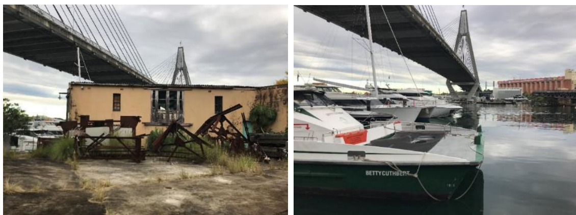
Figure 3.4 Existing buildings on-site (left); view looking north to marina and Bays West (right)
