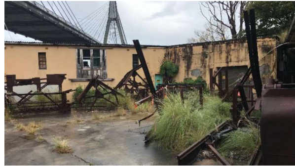
Figure 2.3 1-3 Bank Street, showing concreted courtyard space.
