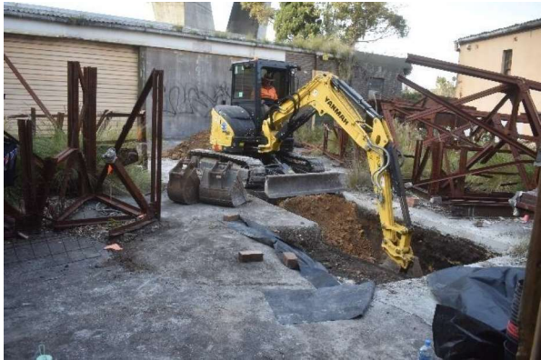
Figure 2.8 Trench 01 mid-excitation, showing spatially constrained nature of 1–3 Bank Street courtyard.
