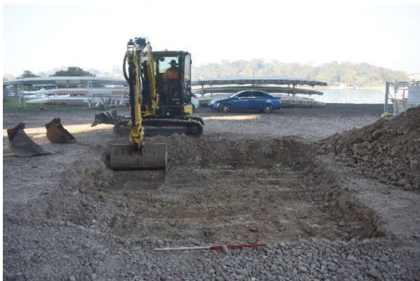
Figure 2.26 Trench 5, start of excavation, showing position within DBNSW compound, facing south.
