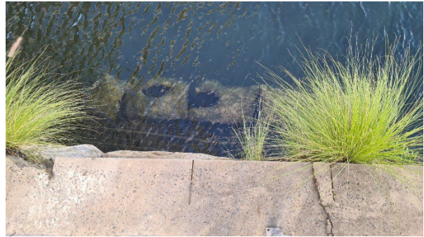
Figure 3.5 Detail of sandstone and metal mesh feature in water below sandstone seawall. View to southwest.
