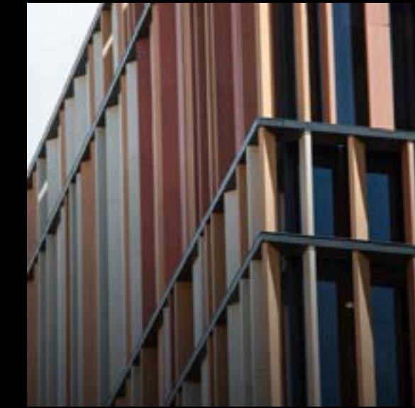
Baguette ventilated terracotta system Tempio
