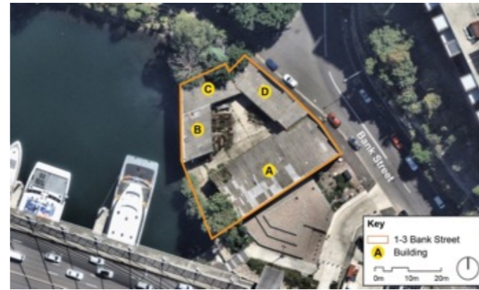
An overview of 1-3 Bank Street, showing the buildings in the site. (Source: Nearmap with GML overlay)
