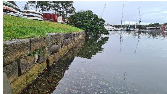
Figure 2.48 Detail of the sandstone seawall of the empty gravel lot.
