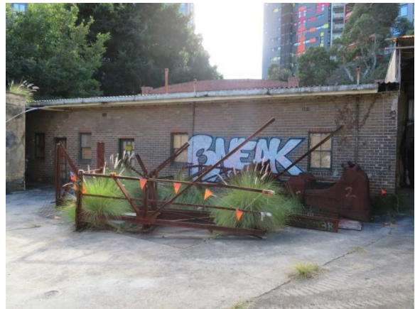
Figure 2.28 Building D from the internal courtyard.
