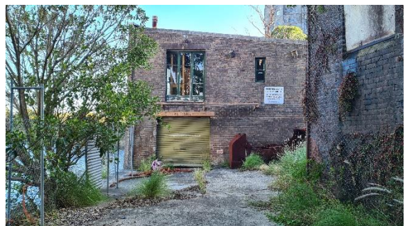
Figure 2.30 Building B from beside the water, showing the 'Workshop' sign and timber rack over the roller door.
