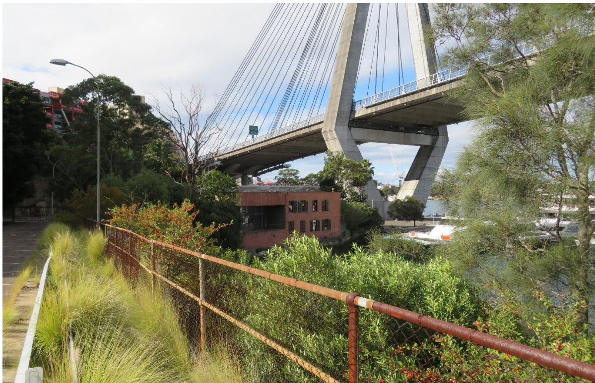
Figure 2.52 View 4 of the waterside elevations of the buildings at 1–3 Bank Street from Glebe Island Bridge.
