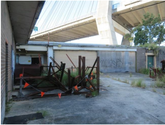
Figure 2.25 Building A from the internal courtyard.
