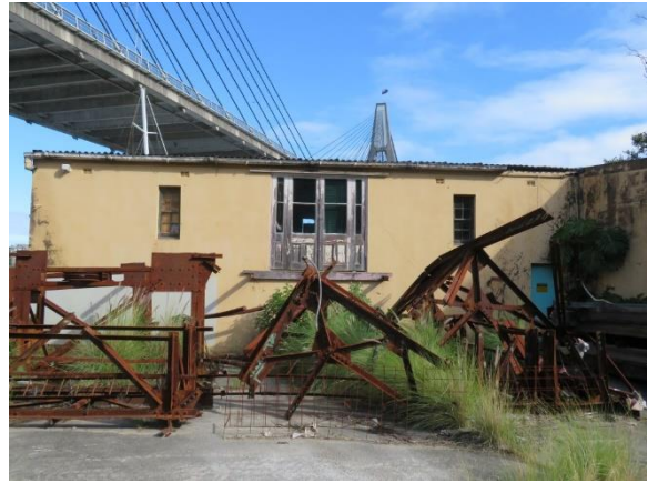
Figure 2.26 Building B from the internal courtyard, showing the goods door.
