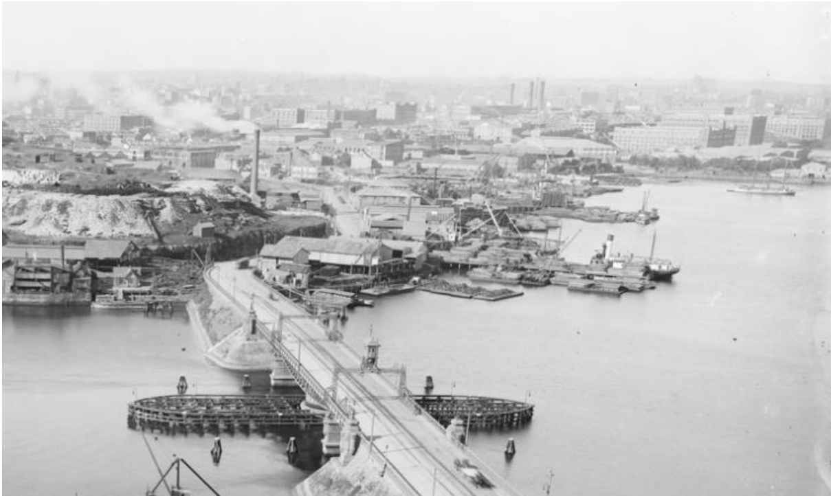
Figure 2.8 Detail of an aerial from Glebe Island Bridge to Pyrmont c1927. (Source: State Library of NSW [FL383183])
