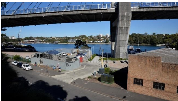
Figure 2.41 The eastern pylon of Anzac Bridge, and Blackwattle Bay Marina.
