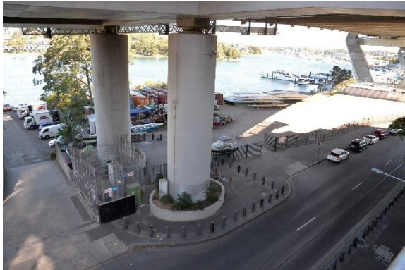
Figure 2.45 The two Anzac Bridge piers on the southeast boundary of the site.
