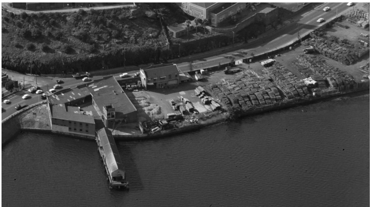
Figure 2.11 Oblique aerial of the site in 1963 by Clive Kane, showing 1–3 Bank Street intact and 5 Bank Street used for storage. (Source: SLNSW [FL14291296])
