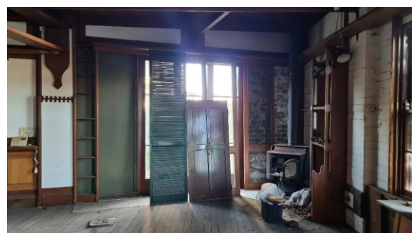
Figure 2.36 Room B1 continued, showing the southern goods door.
