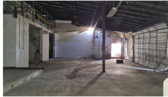
Figure 2.32 Room A7 of building A, the main warehouse space.
