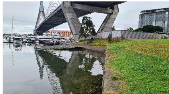
Figure 2.44 View to the reclaimed land of the eastern pylon and the boat ramp.
