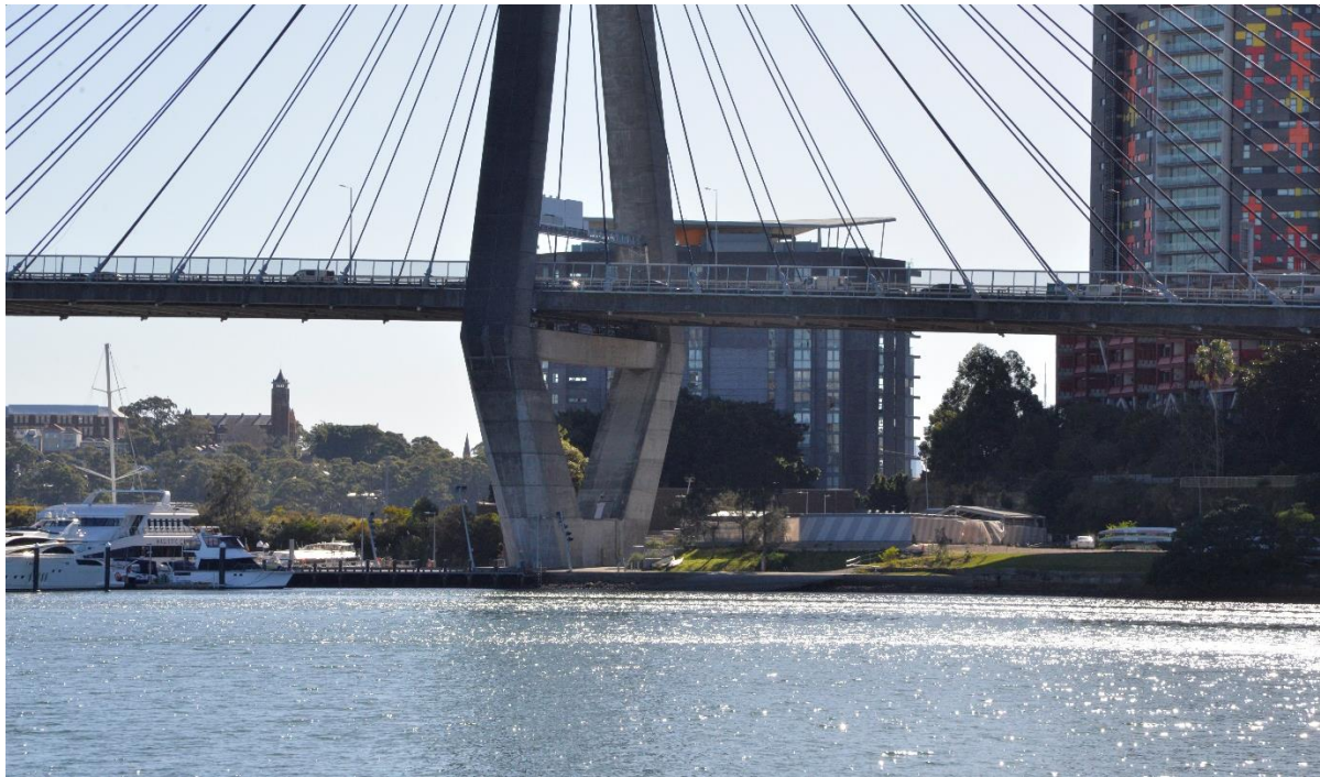
Figure 2.51 View 3, oblique view to the site from the University of Sydney Boatshed in Blackwattle Bay.
