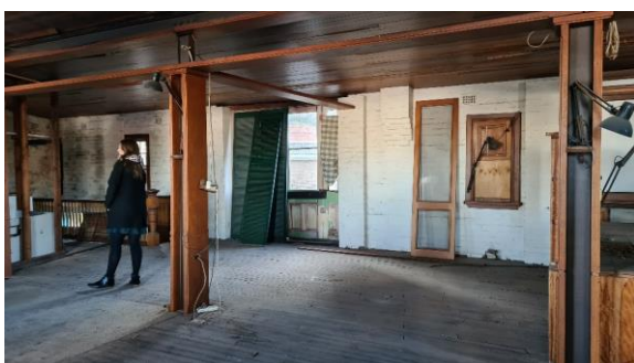
Figure 2.35 Room B1 of building B, showing the modern timber joinery.
