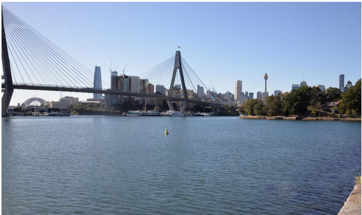
Figure 2.50 View 2, distant view to the site from Pope Paul IV Reserve on Glebe Point, broadly representative of the views from Rozelle Bay.
