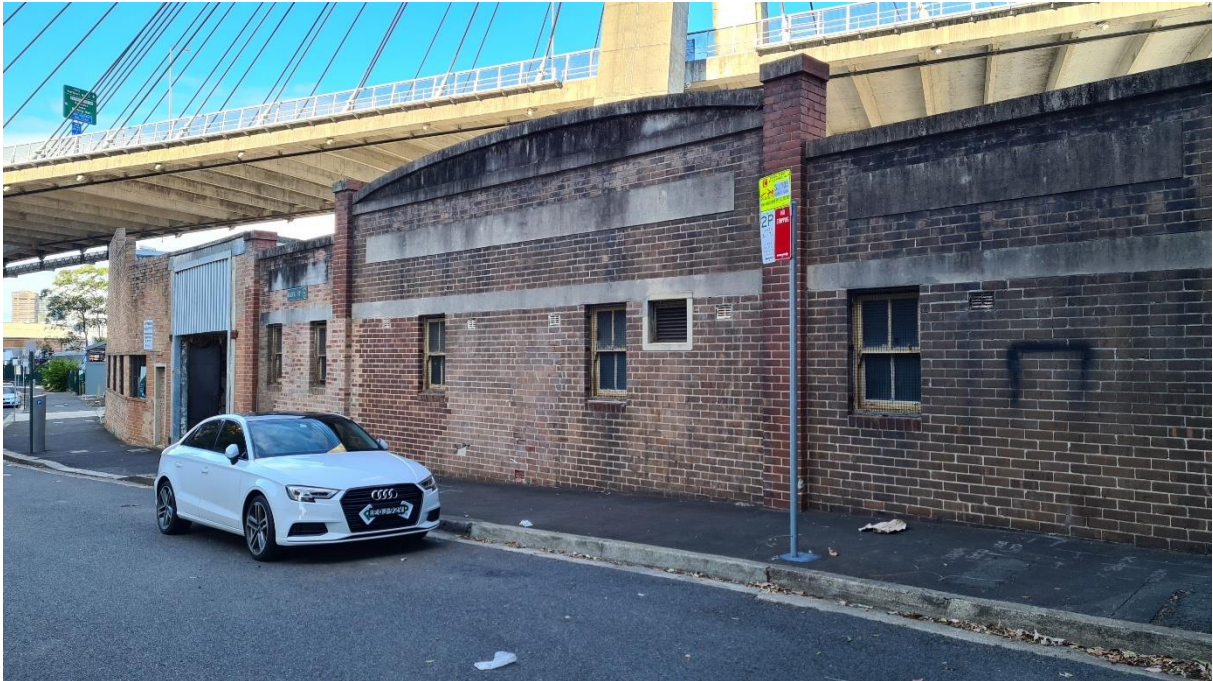
Figure 2.53 View 5 of the buildings at 1–3 Bank Street from Bank Street.
