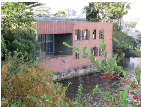
Figure 2.23 The west elevation of buildings B and C.
