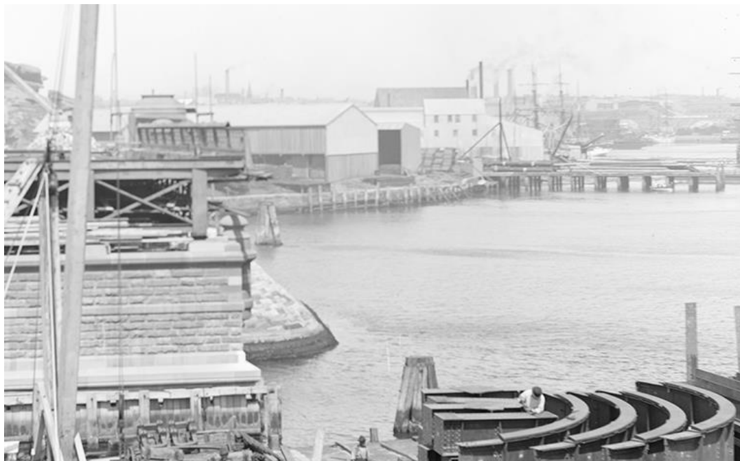
Figure 2.7 Detail of an image of the construction of the Glebe Island Bridge turntable c1899–1902, showing the Augeson & Co timber yard buildings and wharf in the background. (Source: State Records of NSW [AF00257768])
