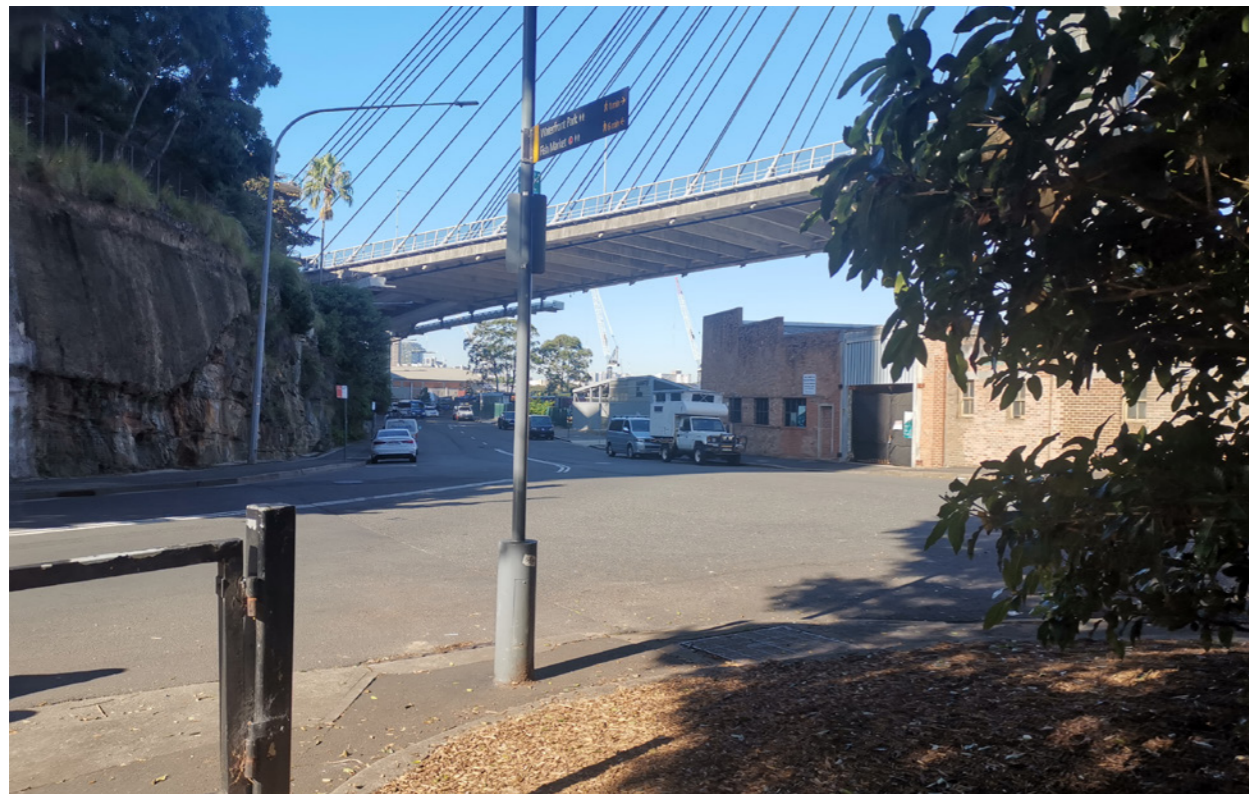
Figure 37: Existing northwest views of the site. Source: Architectus
