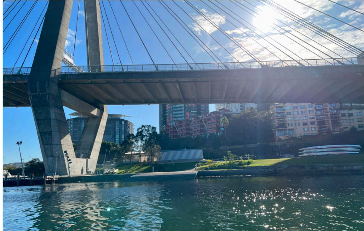
Figure 39: Existing southern views of the site (from Blackwattle Bay)
