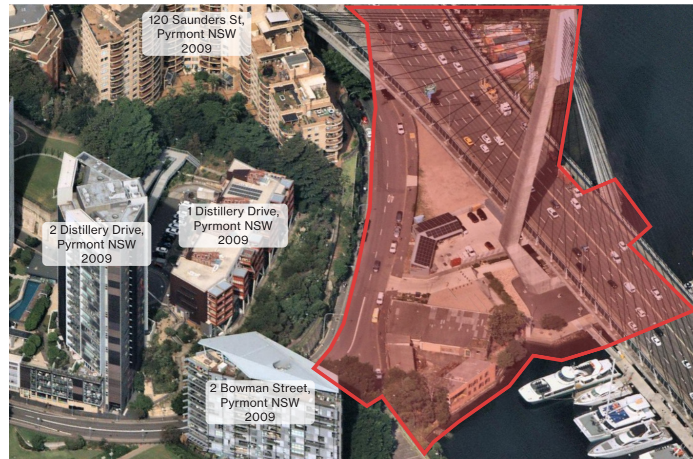
Figure 24: Birds-eye view of site context from north
