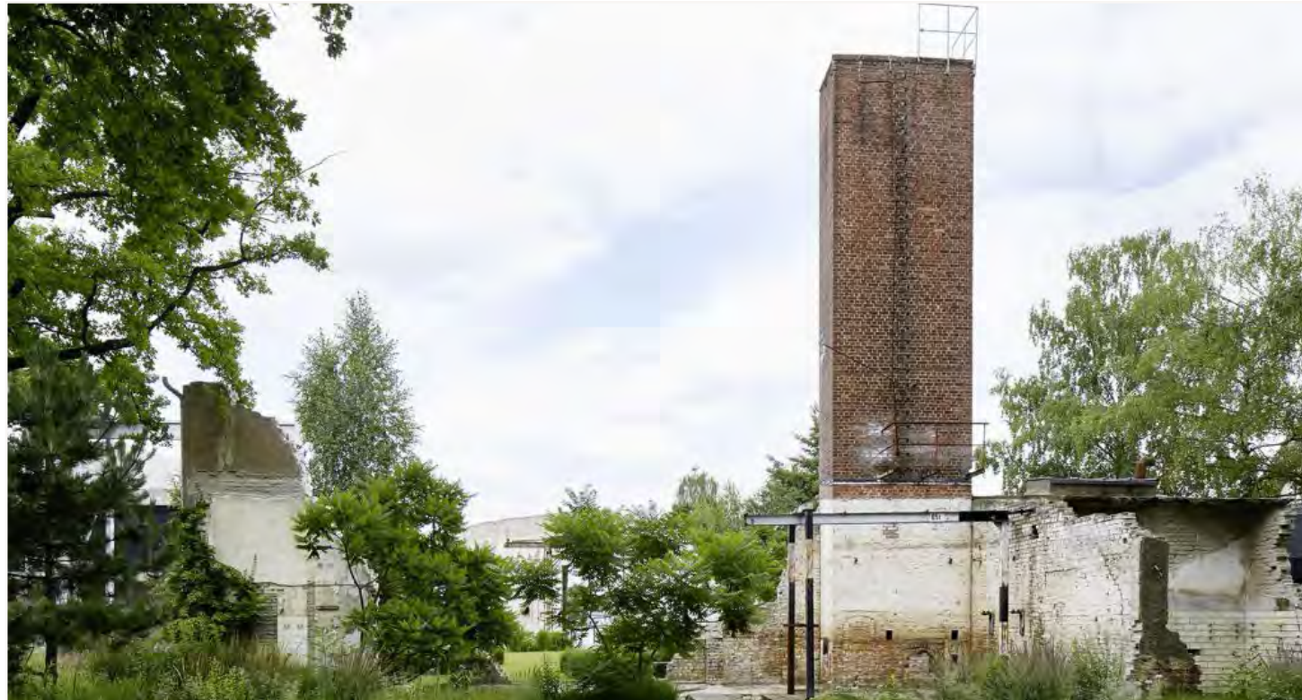
Retained walls and chimney with new planting and concrete paving
