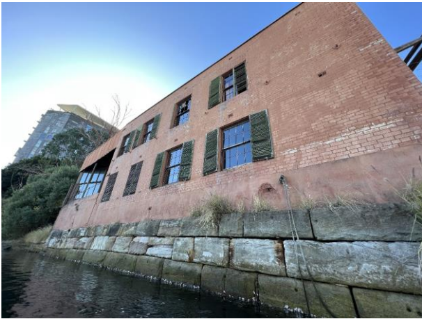
Vertical sandstone block seawall northern side of Anzac Bridge (walls to remain).
