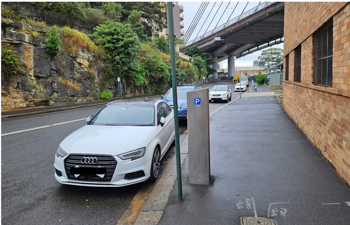
Figure 8 Existing Bank Street footpath
