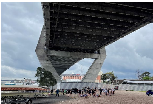
Figure 8 The southern pylon of Anzac Bridge Source: Oculus (2022)
