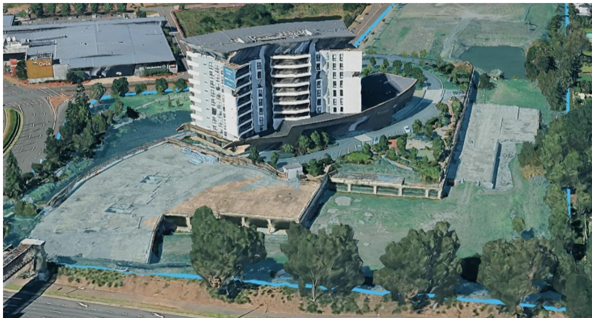
Figure 10: Existing Structure on site
