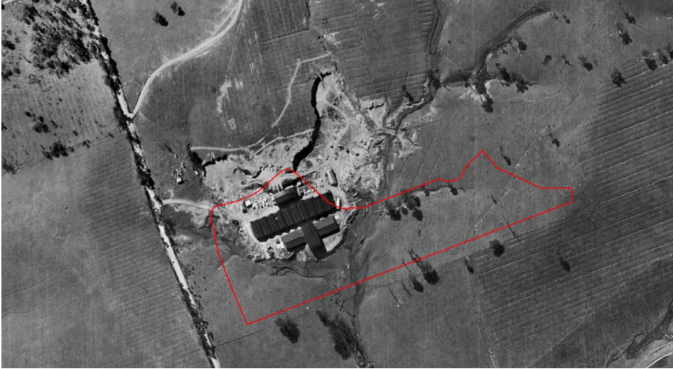
Figure 7 1965 aerial, note construction of large industrial buildings and associated quarrying activity.
