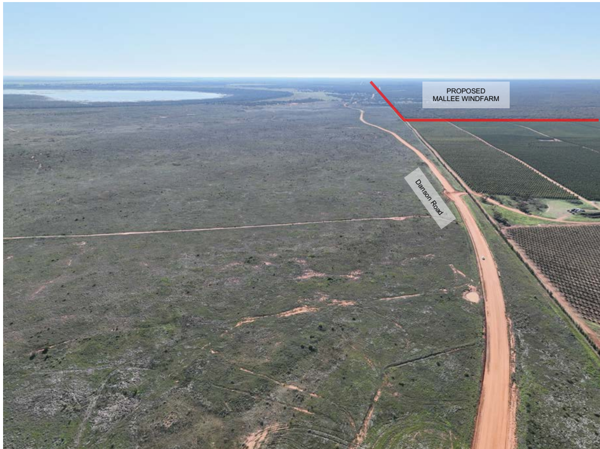
Figure 31 - Danson Rd Looking North
