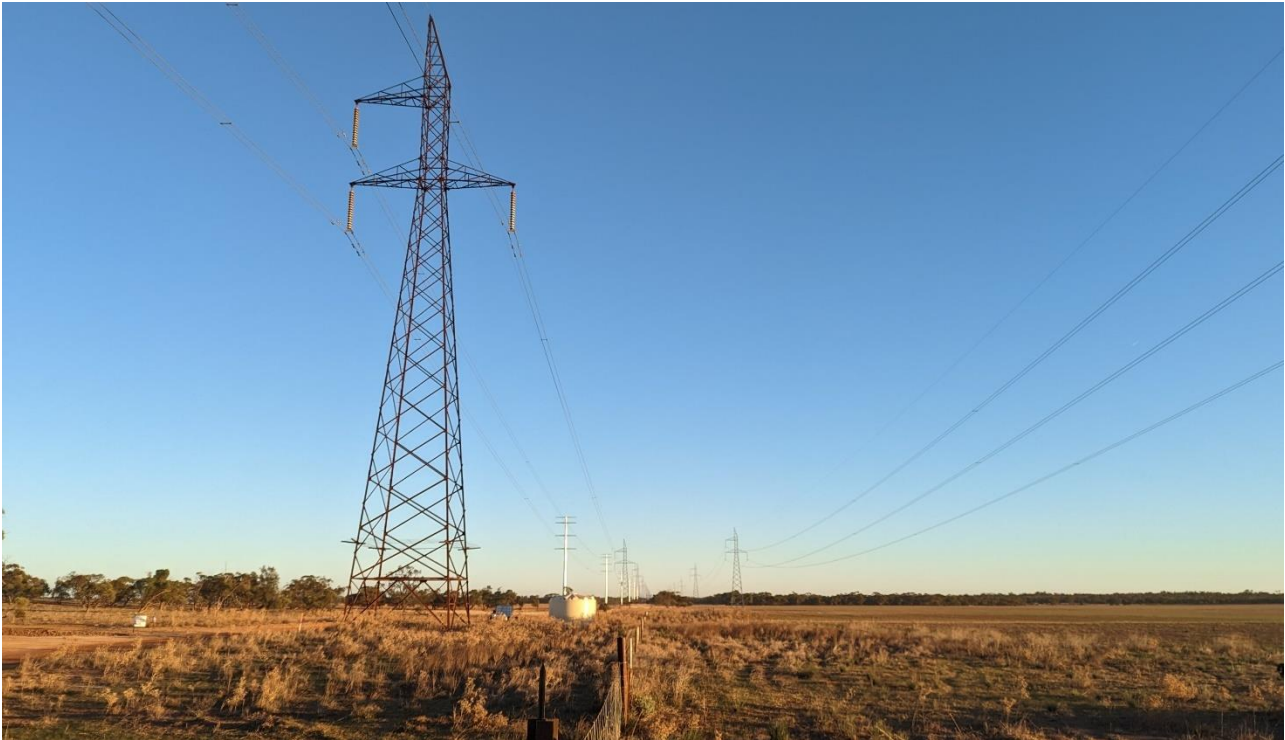
Figure 3.11 Typical Overhead Transmission Line Configuration
