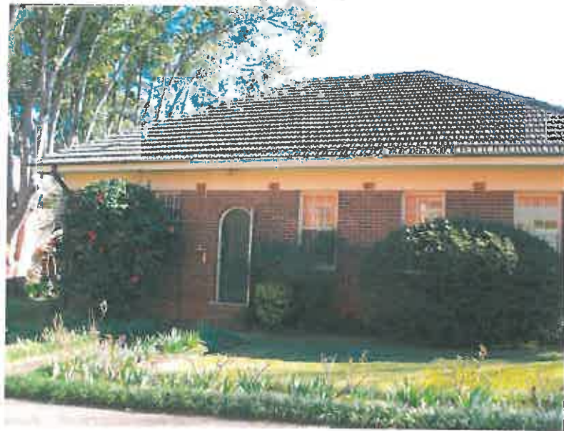
Figure 6: Existing hospital building to be demolished
