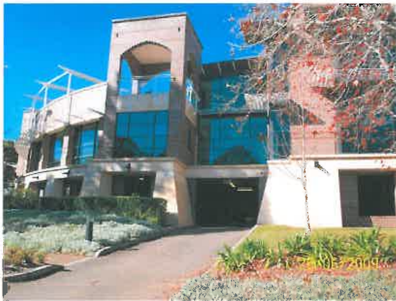
Figure 1: Existing library building
