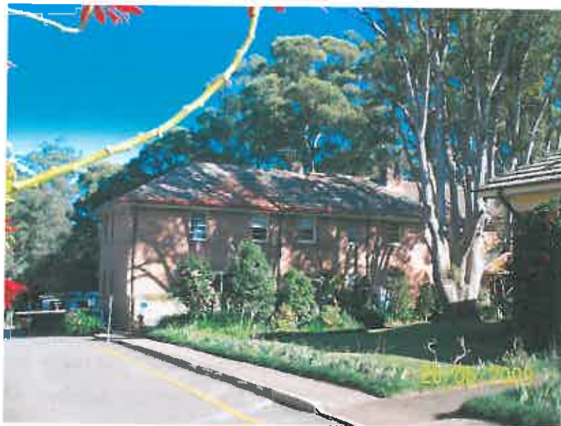
Figure 7: Existing Nancy Jobson building to be demolished
