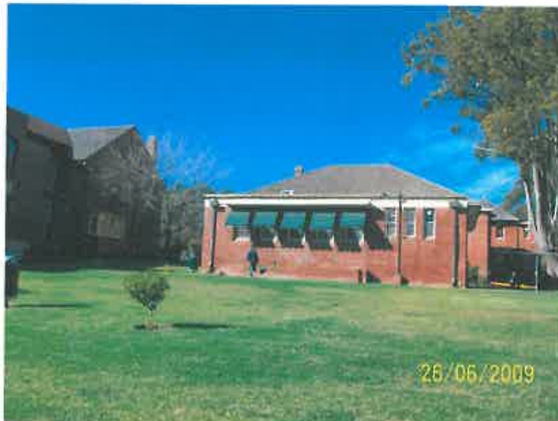
Figure 2: Existing library and location of proposed Senior Learning Centre (existing hospital building to be demolished)
