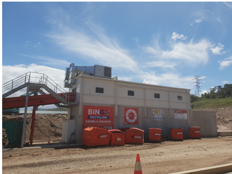
Figure 1: Pick-station constructed at 50 Wylie Rd, Kemplra Grange
