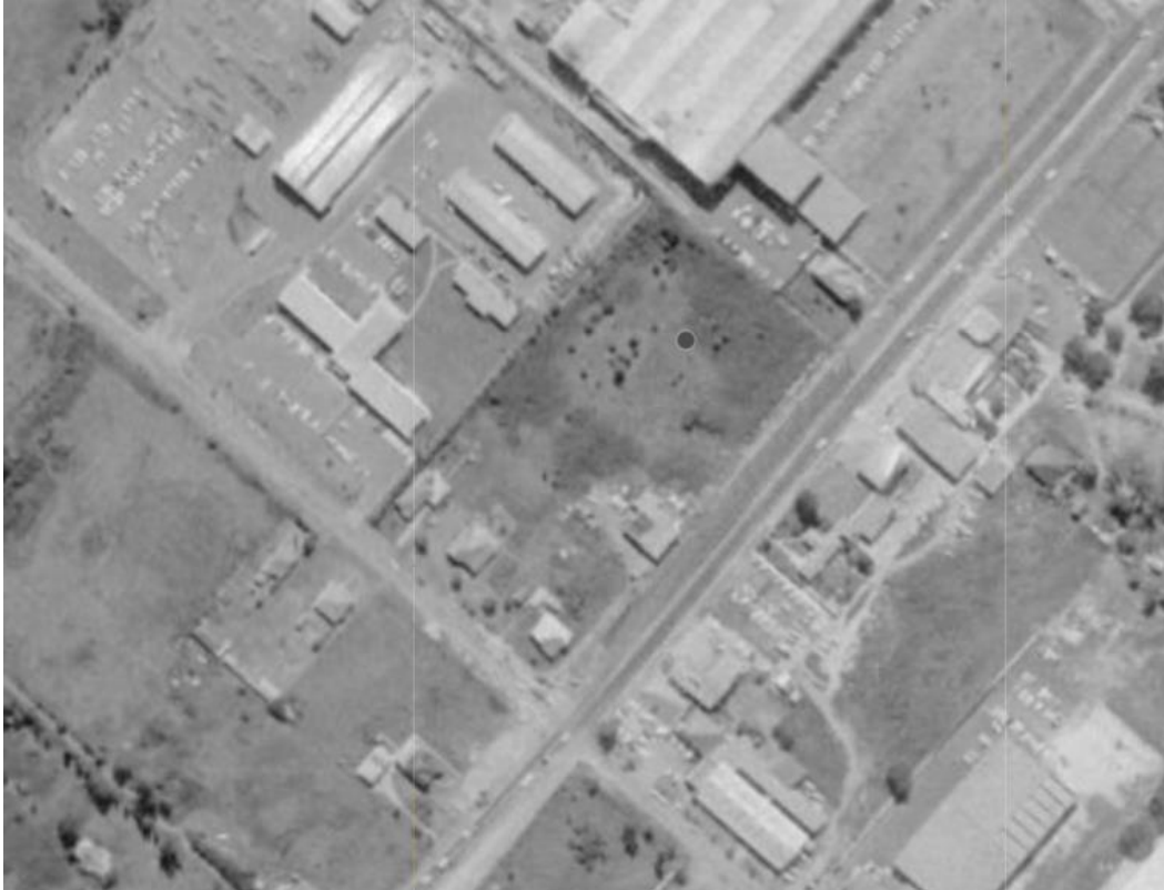
Figure 6: 1970 area aerial image of the study area 35 Waterloo Road, Macquarie Park (Historical Imagery Spatial Services)
