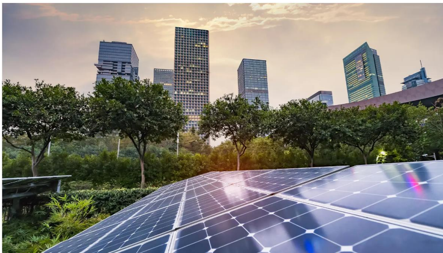
Figure 2: Solar installation example
