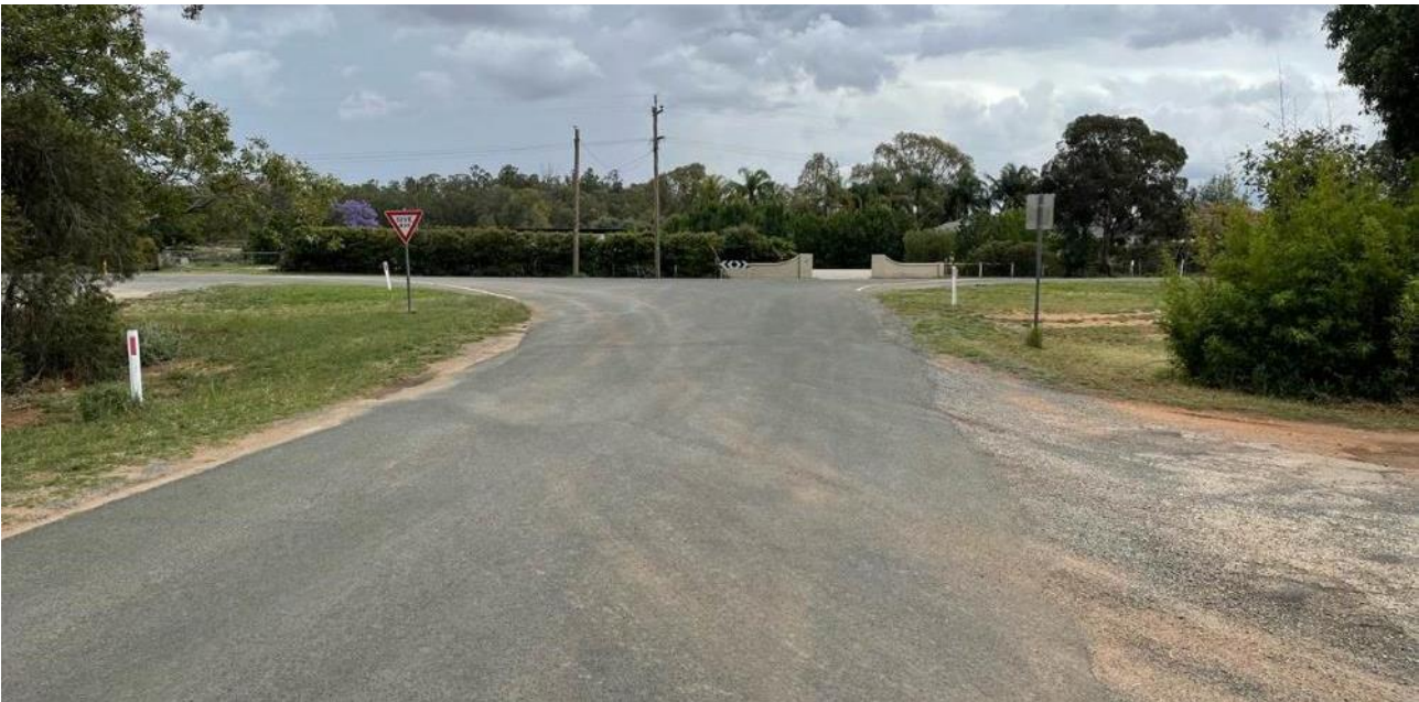
Plate 2.5 Piper Street (looking south towards Sturt Highway)
