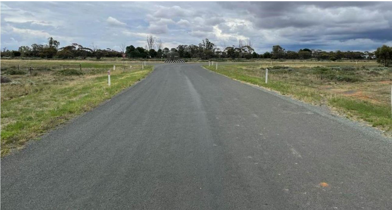
Plate 2.4 McCabe Street (looking west towards Balranald-Ivanhoe Road)
