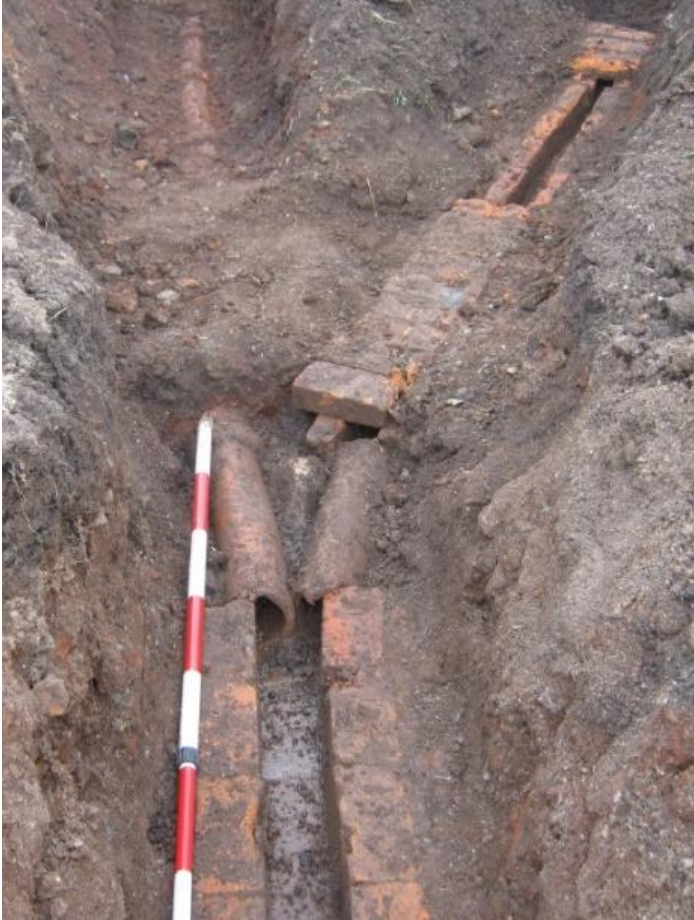
Photo 14 A drainage system incorporating historical and modern drains
