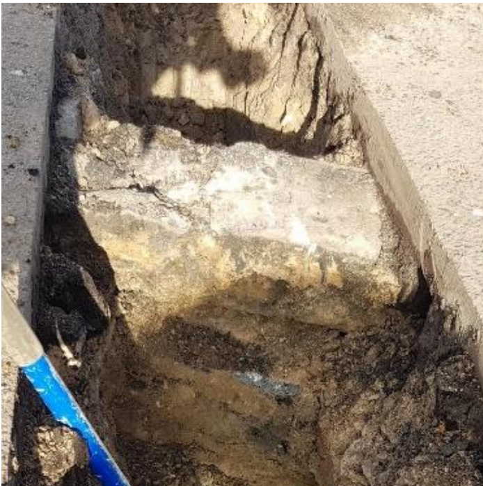
Photo 15 Wall footings (stone/sandstone)
