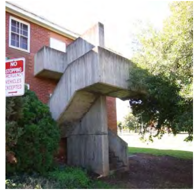
Figure 103 1936 nurses' building exterior showing later fire stairs
