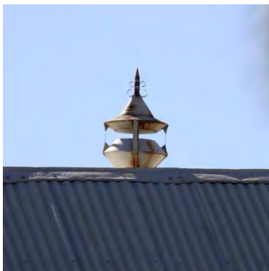
Figure 71 1907 building exterior showing roof ventilator
