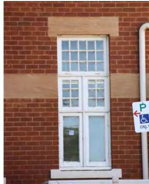
Figure 66 1907 building exterior showing feature windows
