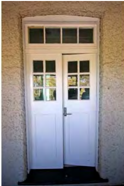
Figure 83 1907 exterior upper floor showing balcony doors
