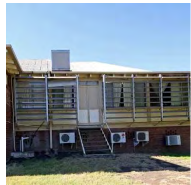
Figure 91 1926 additions to 1868 building exterior showing verandah. The c1970 louvres have not survived well and are now detracting from the building
