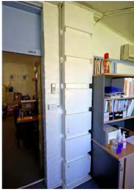
Figure 49 1868 building interior showing original pilaster
