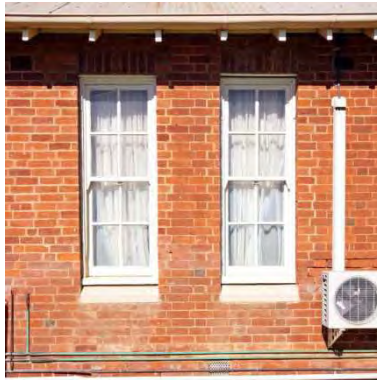
Figure 93 c1890 additions exterior north face showing 1926 windows cut into wall. The discoloured mortar shows where bricks were removed.
