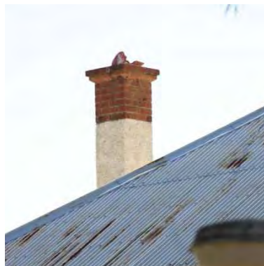
Figure 72 1907 building exterior showing original chimney
