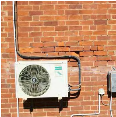
Figure 95 c1890 external wall where the soft bricks are being seriously damaged by air conditioning unit – the units need to be removed
