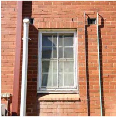
Figure 101 1936 nurses' building exterior showing typical window
