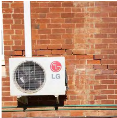
Figure 96 c1890 external wall at junction with 1926 addition where the stronger bricks are not suffering as greatly.
