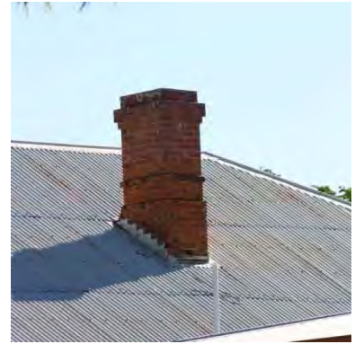
Figure 51 1868 building exterior showing original chimney
