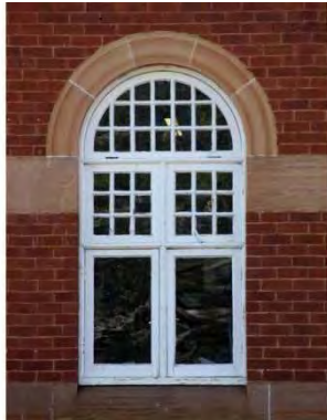
Figure 65 1907 building exterior showing feature windows
