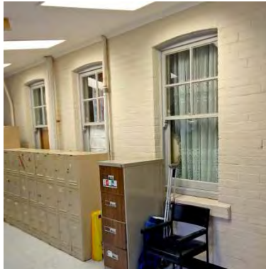
Figure 84 1907 exterior lower floor showing 1907 central wing windows
