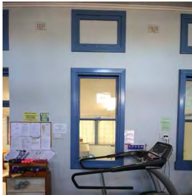
Figure 53 1887/1907 building interior - 1907 windows, possibly modified 1926
