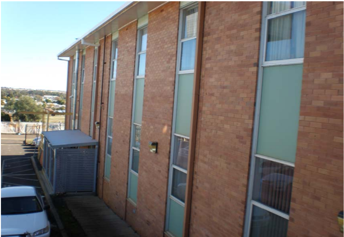
Photo 16/8 - Bonded asbestos window spandrels
