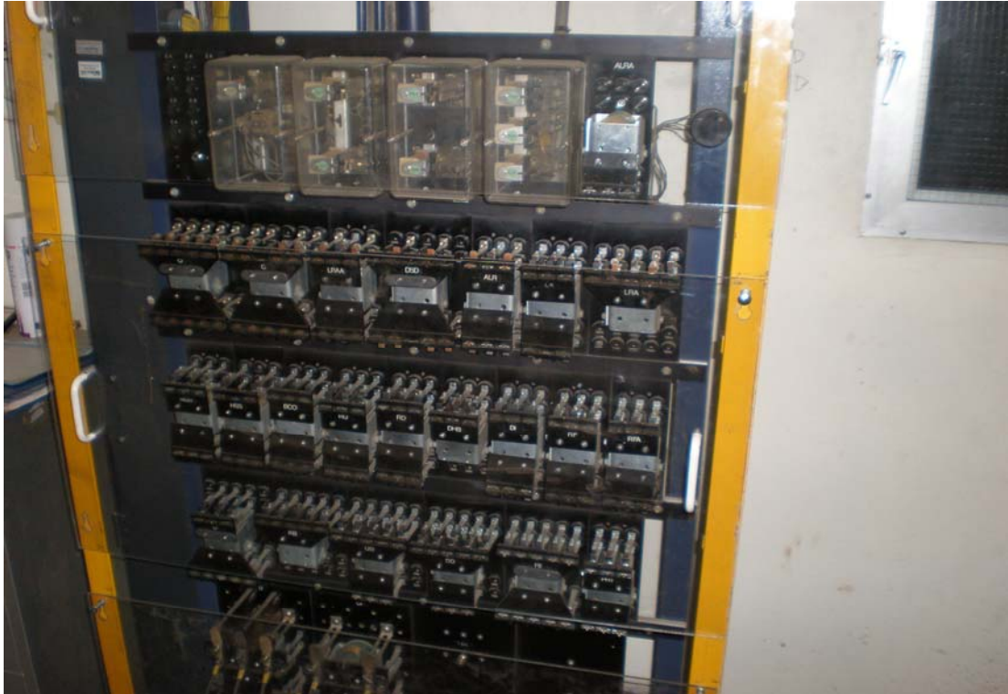
Photo 16/5 - Bonded asbestos backing-board on lift control panel
