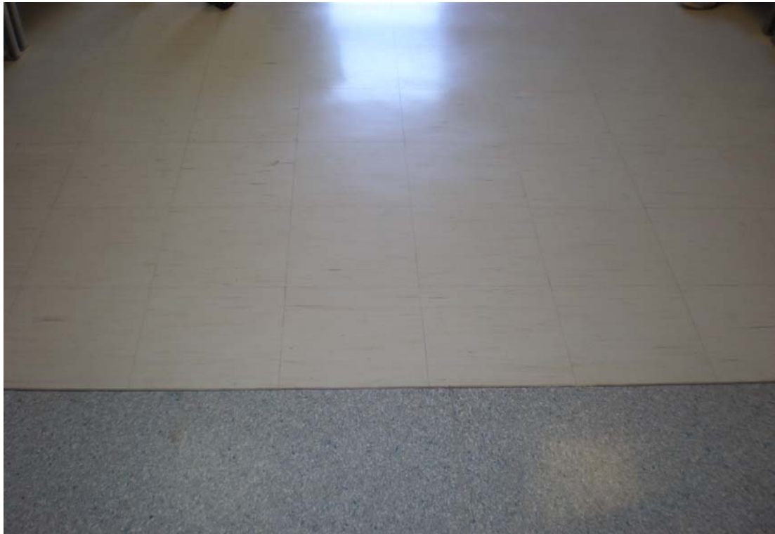
Photo 16/9 - Asbestos vinyl floor tiles
