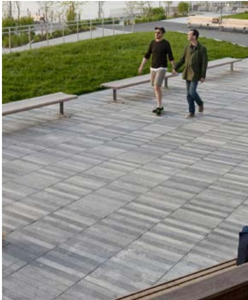
Stack bond concrete paving
