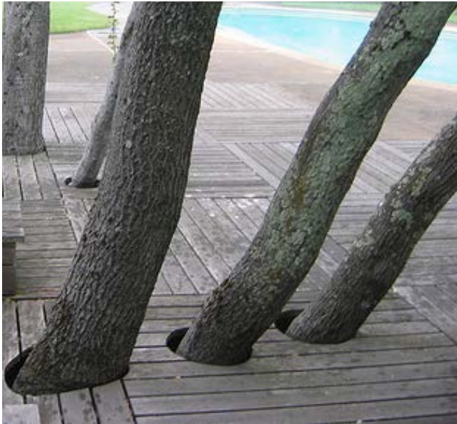
Raised timber platform around existing trees
