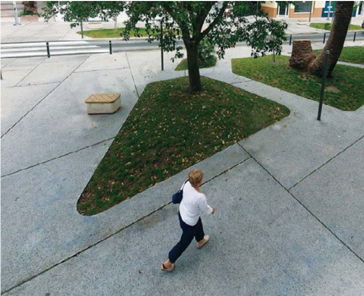
Concrete with saw cuts
