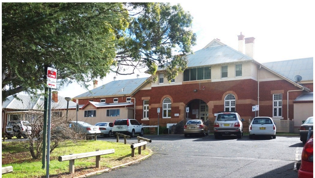
Figure 4 –The 1907 building today – often referred to as ‘the old, old entrance’ to the hospital
