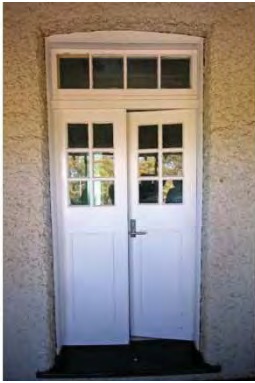
Figure 83 1907 exterior upper floor showing balcony doors
