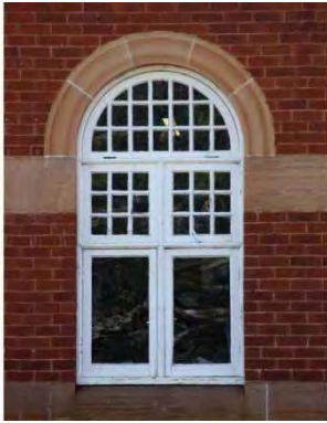
Figure 65 1907 building exterior showing feature windows
