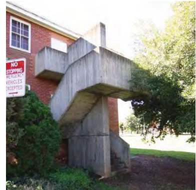
Figure 103 1936 nurses' building exterior showing later fire stairs
