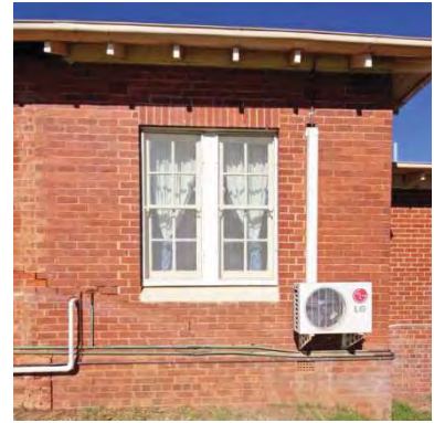
Figure 94 1926 additions exterior north face showing window cut into face c1936
