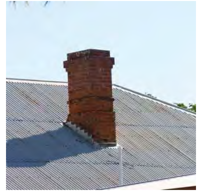
Figure 51 1868 building exterior showing original chimney
