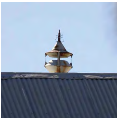
Figure 71 1907 building exterior showing roof ventilator
