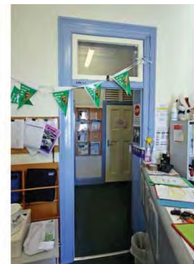
Figure 57 c1890 additions to 1868 building interior showing early intact doorset. All other architraves were stripped out 1926
