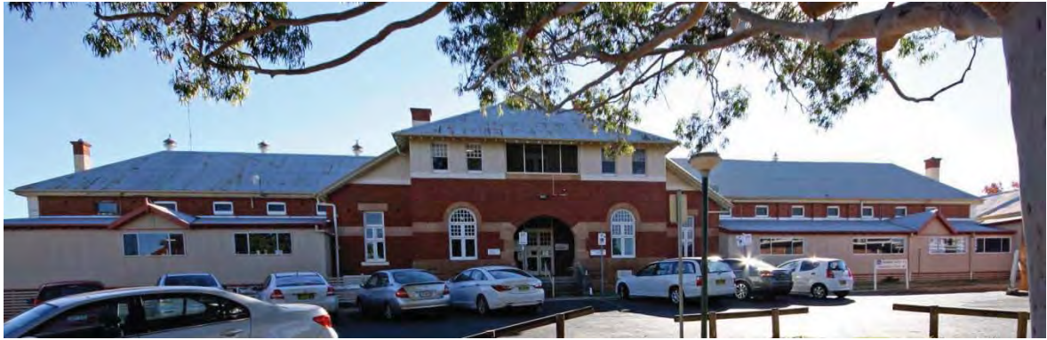
Figure 58 Completed hospital building with 1887, 1907 and 1913 wings. Intrusive infill to verandah greatly reduces the aesthetic impact of the building.
