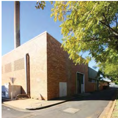
Figure 105 1962 boiler house exterior from south west – this building is to be demolished in the proposed works
