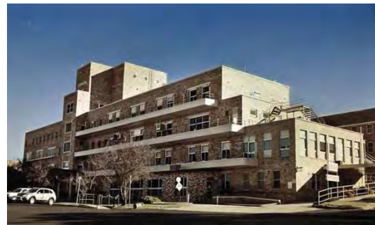
Figure 39 Cowra Hospital was originally designed for Dubbo by Cobden Parkes 1947-1950. 42
