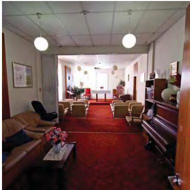
Figure 110 Current chapel room. The first division is the extent of the 1907 fabric. The rear part is made up of 1925 and 1936 fabric. The fireplace was removed c1978.
