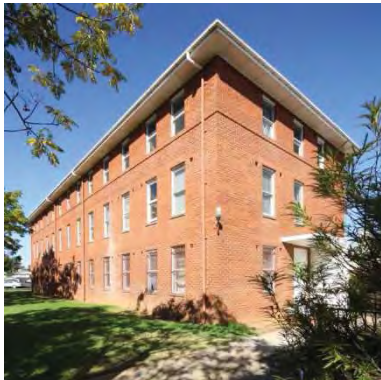
Figure 104 1952 former domestics home exterior from north west – this building is to be demolished in the proposed works
