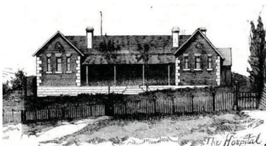
Figure 9 Sketch in newspaper in 1881. Sketch in newspaper in 1881. The artist has added a picturesque 45° pitch to the roof and has made the Georgian windows more like lancets, and the arched highlight more like a trefoil. The artist has changed the pilasters to stepped quoins. Perhaps he was trying to urge the building to be more Gothic. This image is also important for showing the small section of the 1874 building behind the hospital. Town and Country Journal 26.02.1881 p.409
