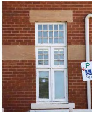
Figure 66 1907 building exterior showing feature windows
