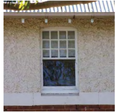
Figure 67 1907 building exterior showing feature windows
