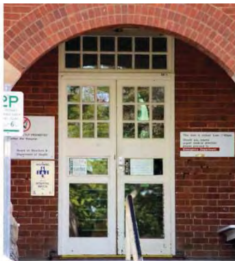
Figure 62 1907 building exterior showing intact main entry door inside brick arch
