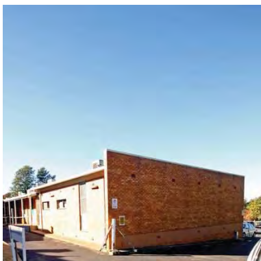
Figure 107 1968 administration building exterior from entry of 1907 building looking towards Myall Street
