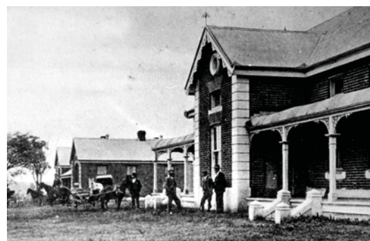
Figure 15 The two buildings formed a streetscape that had a high degree of unity from 1887 to 1907. Macquarie Regional Library Local History
