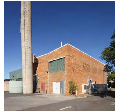
Figure 106 1962 boiler house exterior from north west – this building is to be demolished in the proposed works
