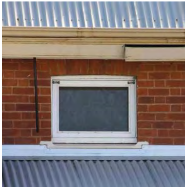
Figure 68 1887/1907 building exterior showing highlight ventilation window – note Flemish bond to brickwork
