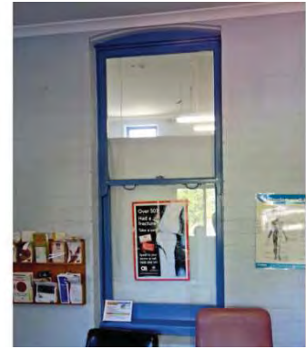
Figure 85 1887/1907 exterior lower floor showing 1907 windows from former verandah side
