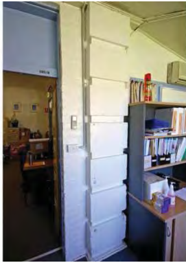
Figure 49 1868 building interior showing original pilaster
