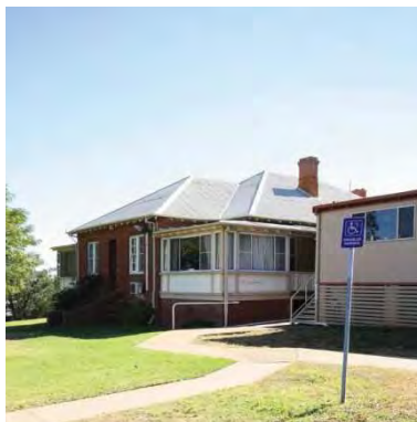
Figure 90 1926 additions to 1868 building exterior showing change to hipped roof
