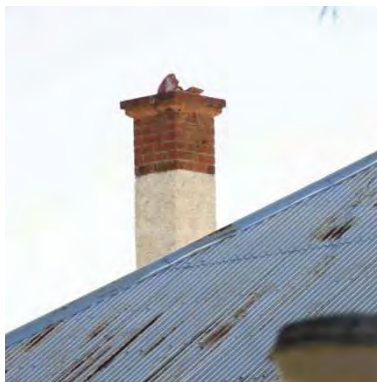
Figure 72 1907 building exterior showing original chimney
