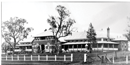
Figure 24 Photo showing the 1913 wing completed. The gable to the left is now the west gable of the partly demolished 1868 building. The transverse gable now facing towards the 1913 wing is the temporary means of addressing the exposed roof space. Incidentally, this is almost the view that could potentially be recovered if the 1966 building was removed and the verandahs reinstated (see below) - Macquarie Regional Library Local History
