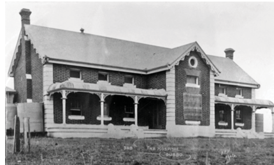
Figure 13 The 1887 Fever Ward building. Macquarie Regional Library Local History
