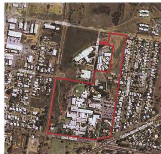
Figure 2 The site boundary of Dubbo Base Hospital. NSW Health Infrastructure
