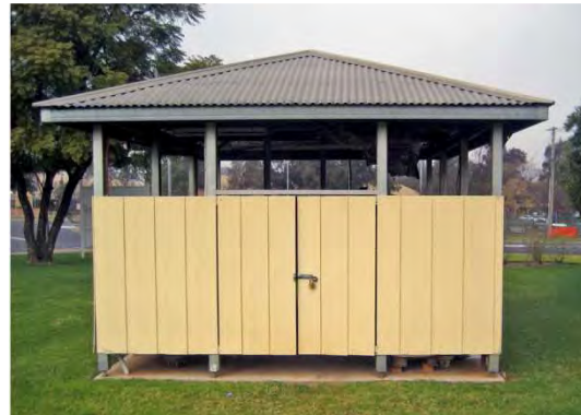
Figure 3 West view of pumphouse
