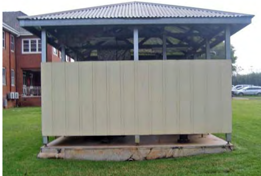
Figure 2 South view of pumphouse with 1926 nurses' building behind
