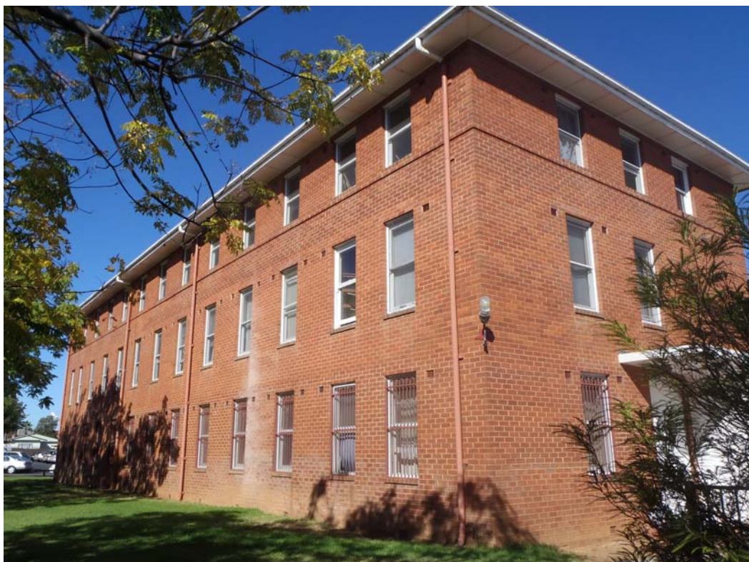
Plate 10: second building to be demolished under current proposal, view south east
