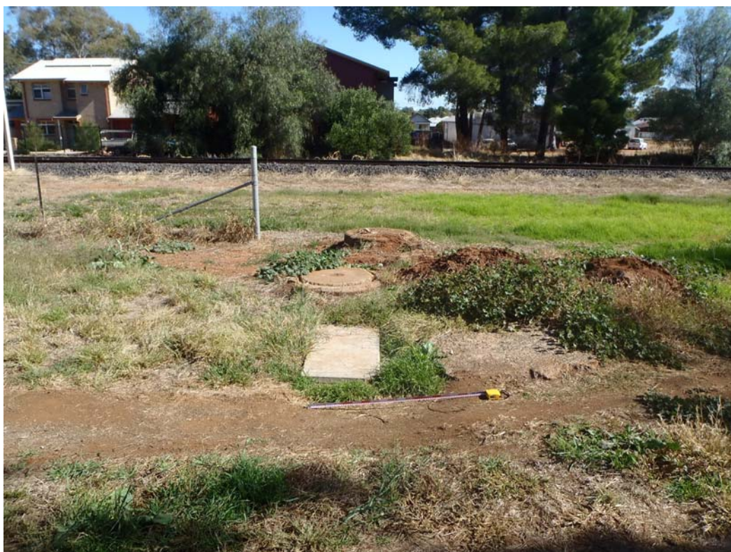
Plate 1: Sewage installation and vehicle disturbance (note railway in the background), view west
