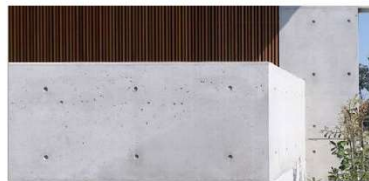
F – OFF-FORM CONCRETE CANDALEPAS ASSOCIATES – KENSINGTON HOUSE
