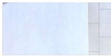
D - WHITE PAINTED CONCRETE CANDALEPAS ASSOCIATES - PINDARI
