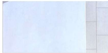
D – WHITE PAINTED CONCRETE CANDALEPAS ASSOCIATES – PINDARI
