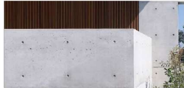
F – OFF-FORM CONCRETE CANDALEPAS ASSOCIATES – KENSINGTON HOUSE
