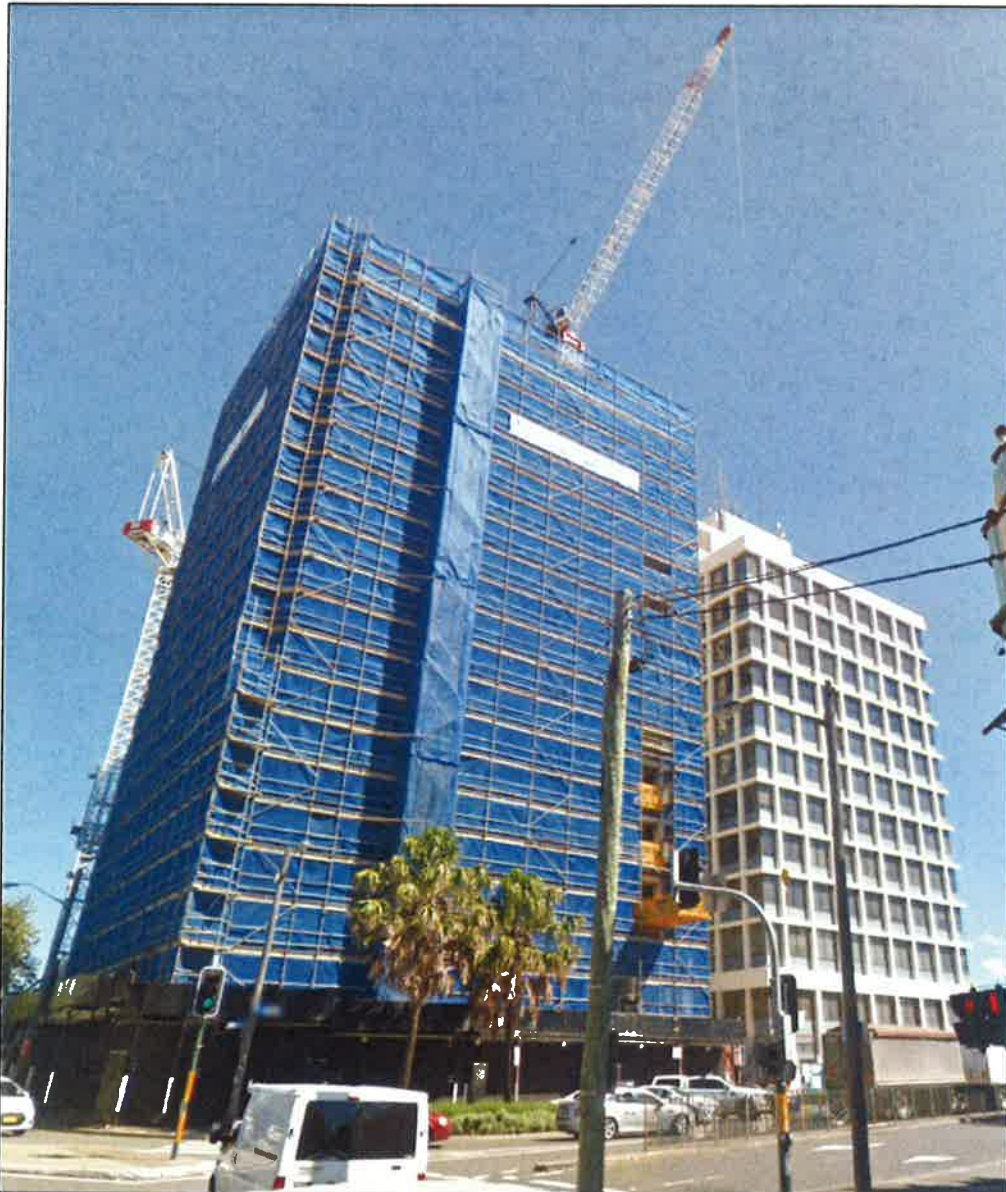
Figure 2: Construction works being undertaken on the site (Source: Google Streetview)
